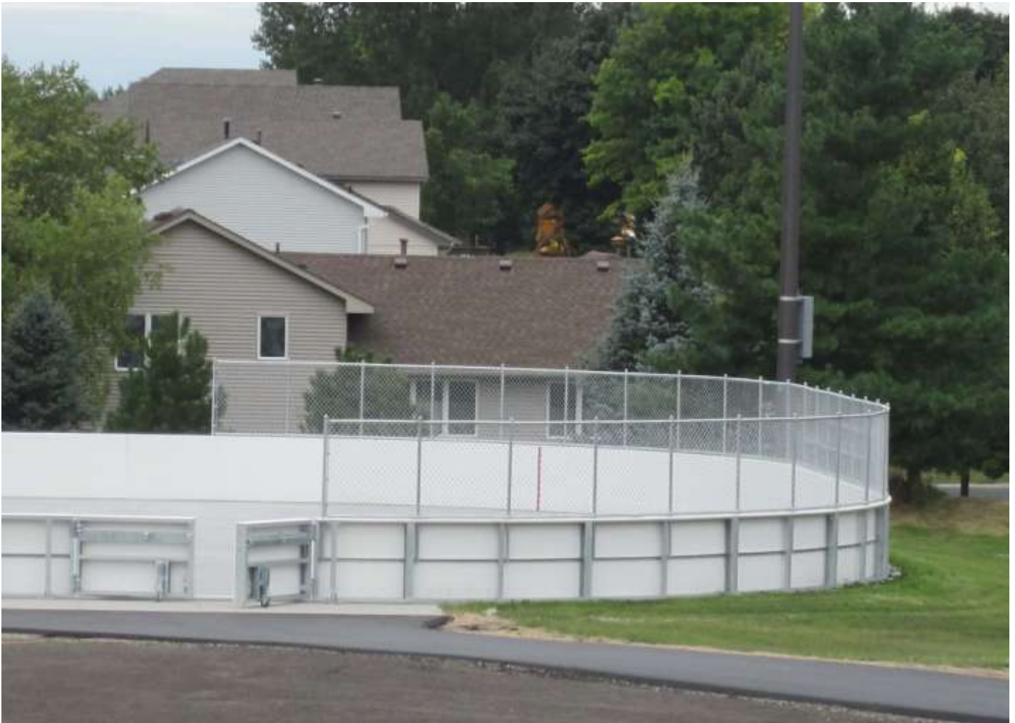
City of Plymouth, Minnesota, Zachary Park. BAP 6.0 Steel Frame Dasher Board System built and installed white fiberglass facing and kickplate, white HD UV polyethylene caprail and chain link fence on both ends.
