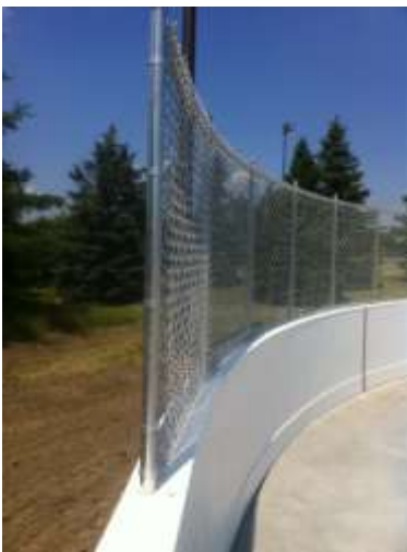
City of Plymouth, Minnesota, Zachary Park. BAP 6.0 Steel Frame Dasher Board System built and installed white fiberglass facing and kickplate, white HD UV polyethylene caprail and chain link fence on both ends.
